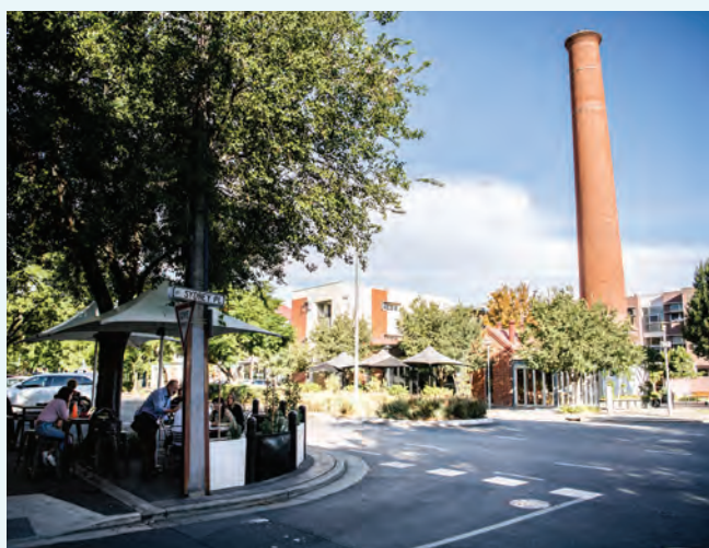
Former City Destructor Complex Heritage Adaption
